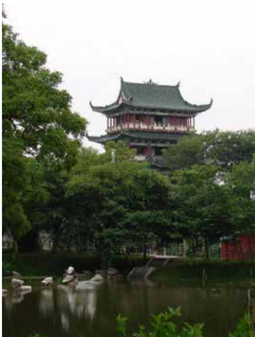
The Bajing Pavilion in Ganzhou, Jiangxi province, China.
